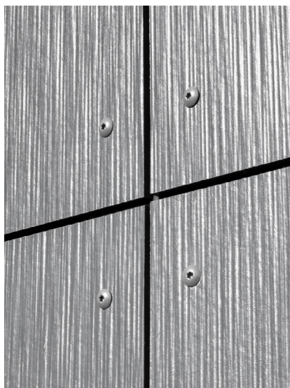
Hardie® Panel Screw Fixing
